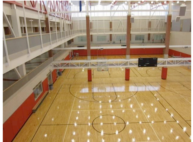
Five Court Gymnasium, with truss support for Basketball Goals
