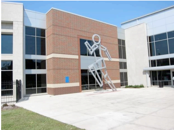
Exterior entry plaza, with significant art work
