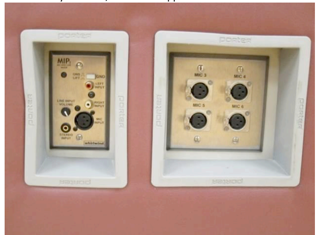
Patron controlled access to sound systems in MP Room, complete with 1/8" iPod connector inputs. Very user friendly.
